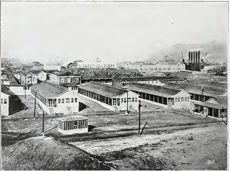
FIG. 101.—Cantonment wards. The first to be erected at General Hospital No. 2.
